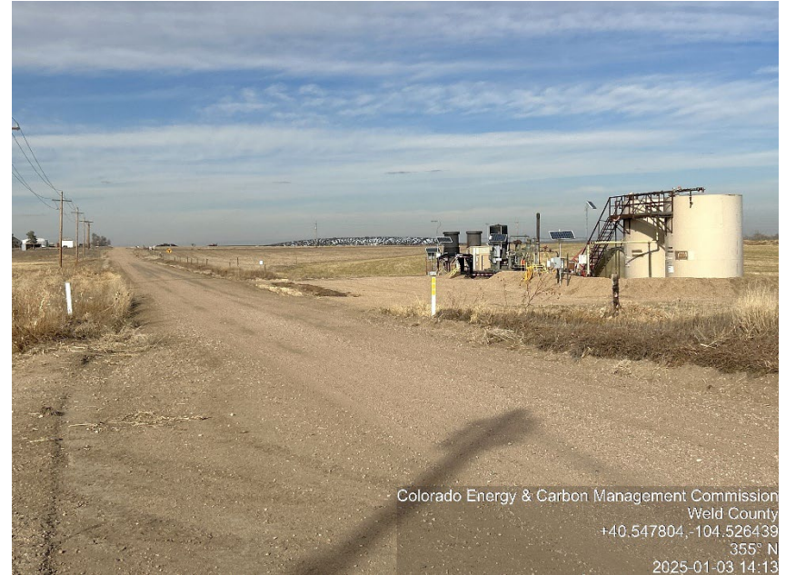
Photo #4 Wilson 4-26, 3-26 Battery site Inactive | Shut-down Battery entrance
