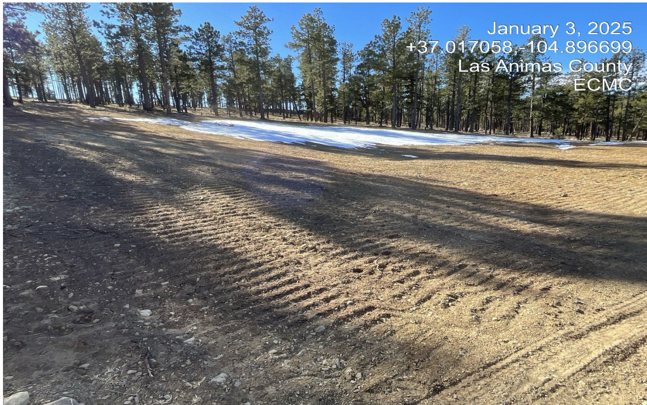
Photo 2. The pit has been backfilled and reclaimed. Soils have been tracked for temporary stabilization.
