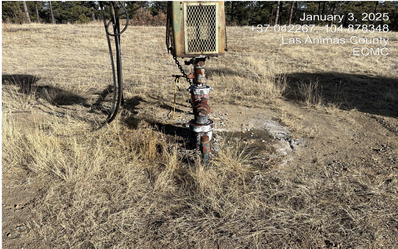
Photo 2. There is a drip leak at the wellhead.
