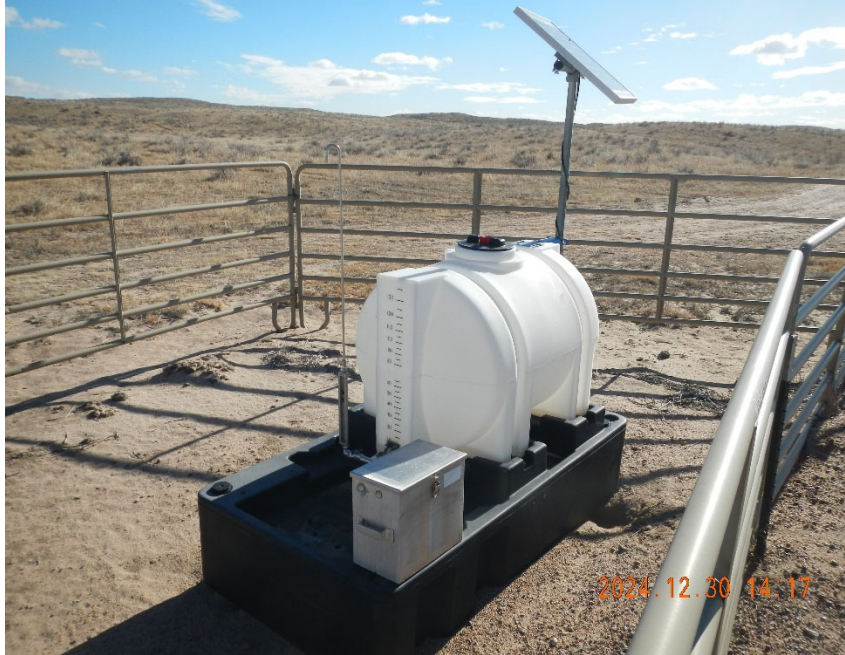
3. View of chemical tank and pump on secondary containment.
