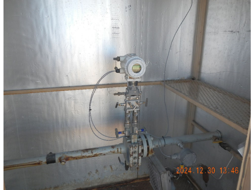
6. Gas meter inside meter shed.
