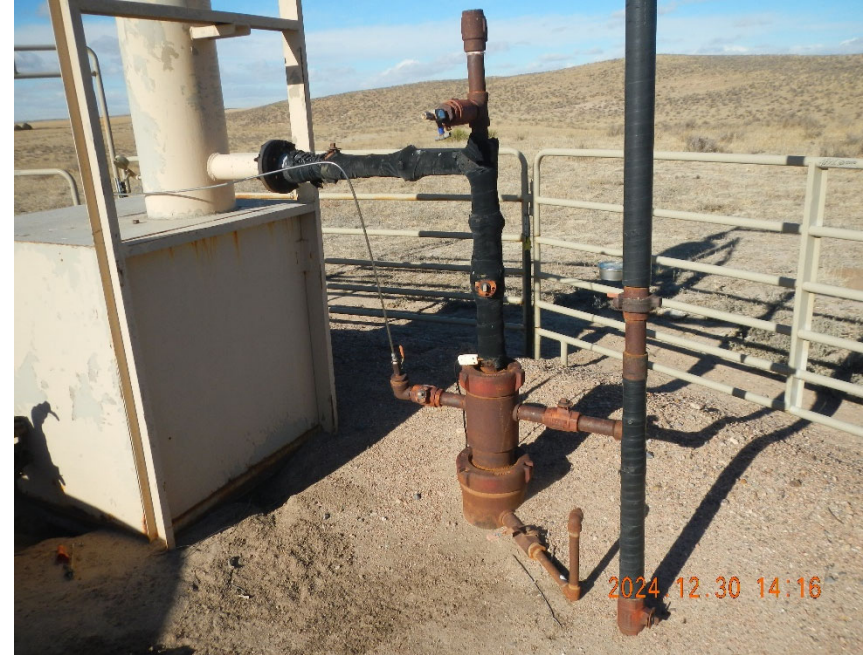
2. View of wellhead and vertical separator.
