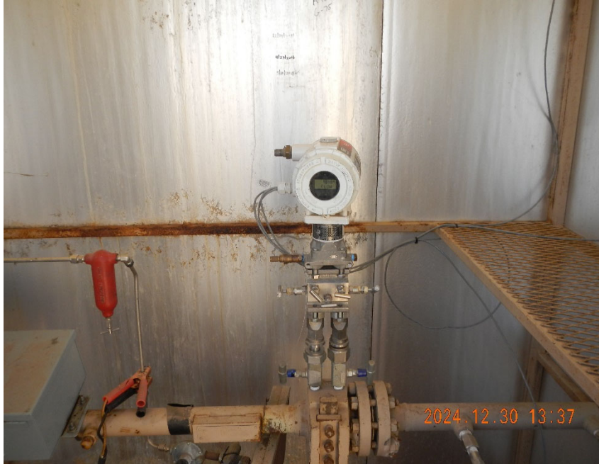
5. Gas meter inside meter shed.
