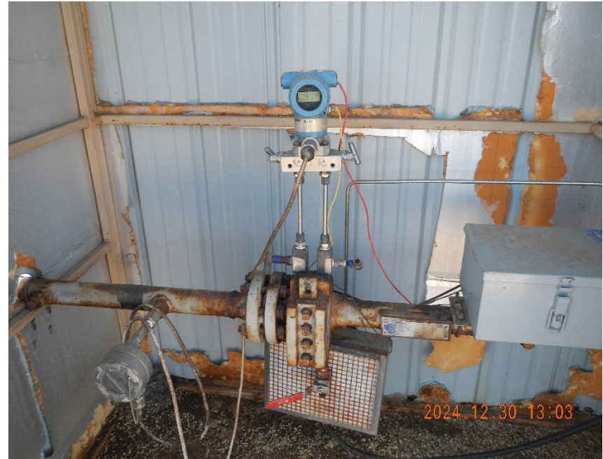
4. Gas meter inside meter shed.
