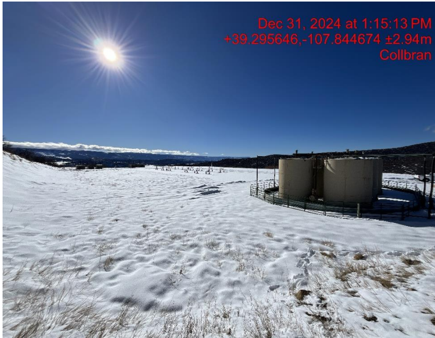
Photo # 1800 NE corner of location
