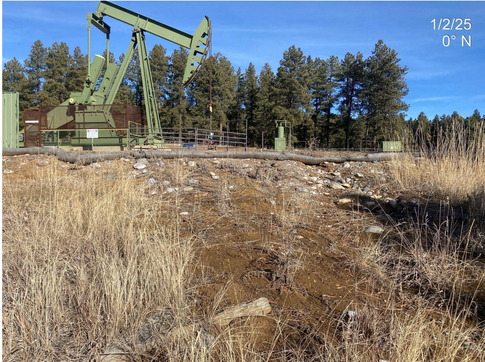
Photo 3. Failing BMPs is leading to sediment transport into the southern interim reclamation area.
