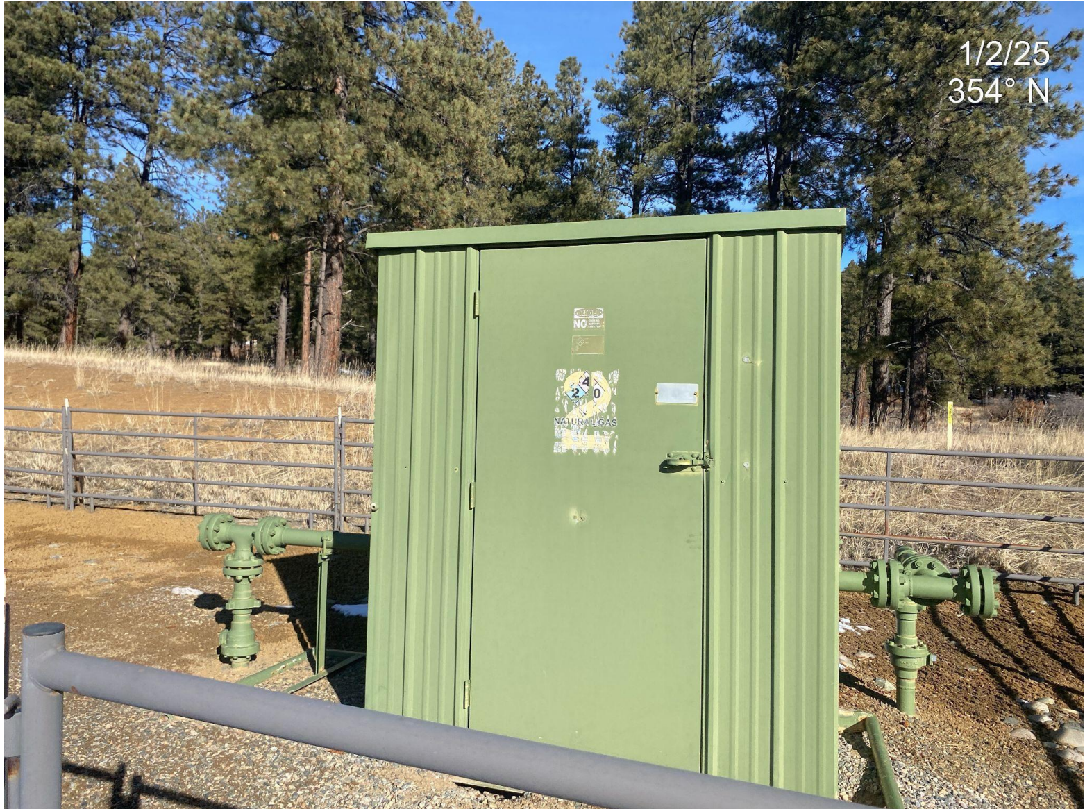
Photo 4. Sign/placard at separator has deteriorated and is no longer legible.
