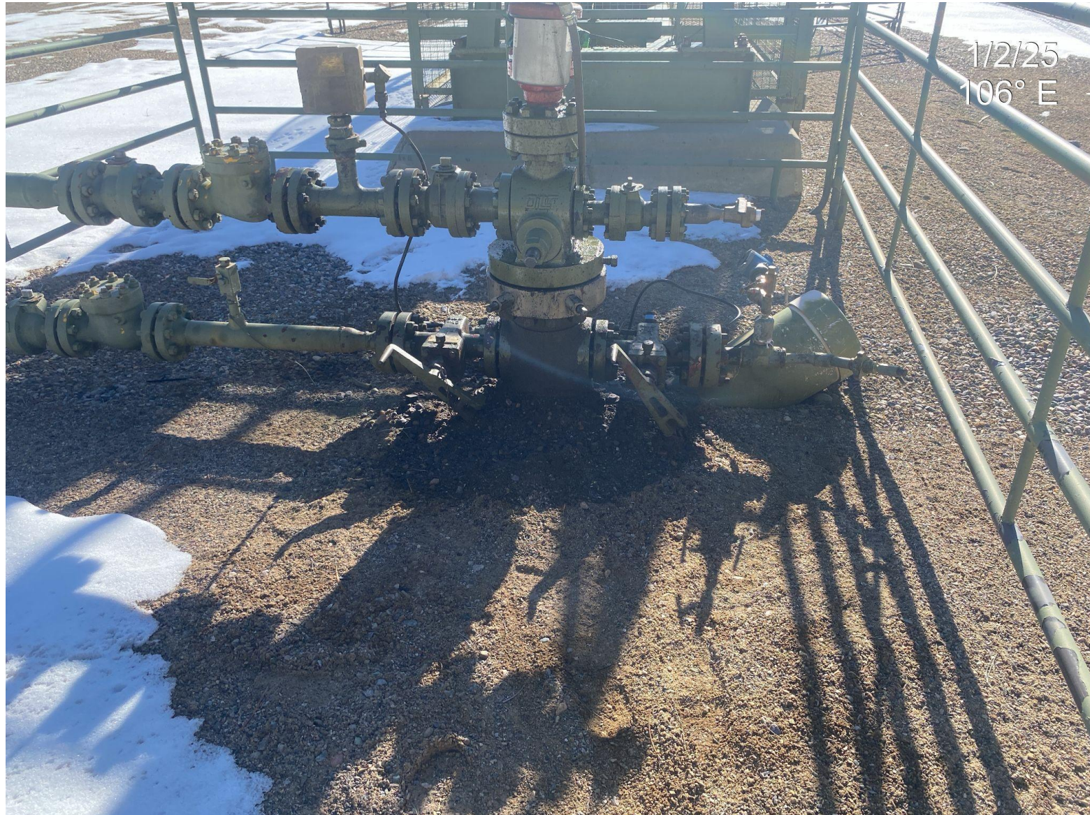
Photo 3. View of stained soils around well head.
