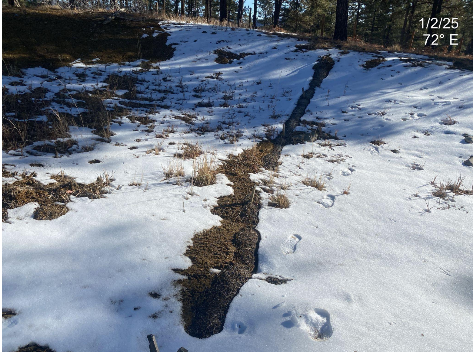
Photo 2. Stormwater BMP/wattles in the eastern portion of the disturbance are filled with sediment and need maintenance.
