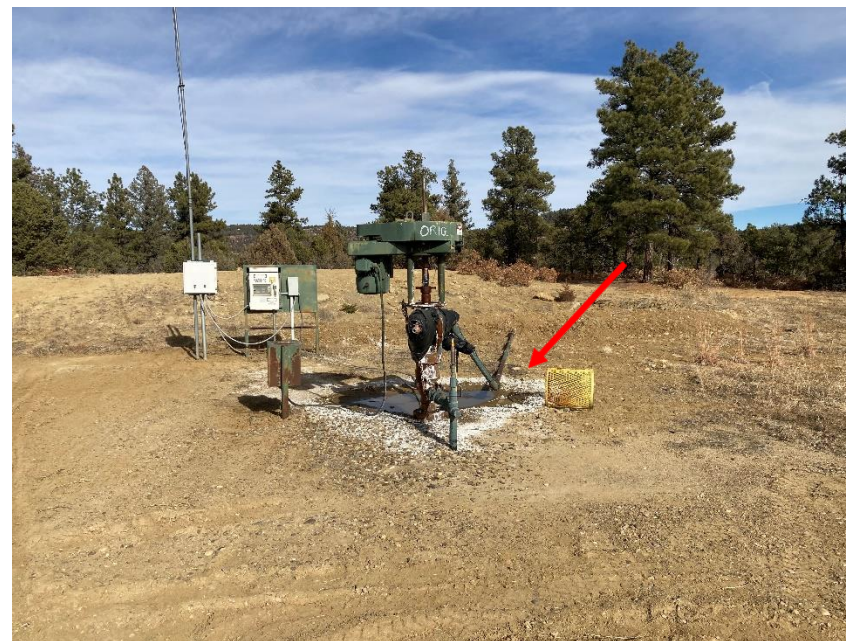
Photo 2 – Original wellhead, Packing leak observed at the time of inspection, White stained soils
