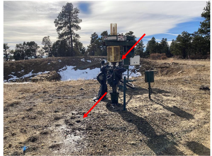
Photo 6 – 41-30 Tr wellhead, Leaking packing
