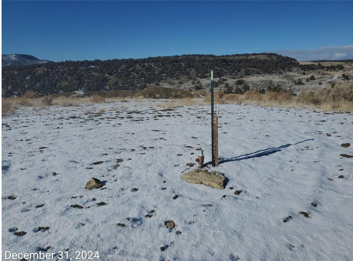
**Photo 3:** Photo shows riser equipment remaining on the north end of the Location. Riser equipment requires removal pursuant to 1004.a requirements.
