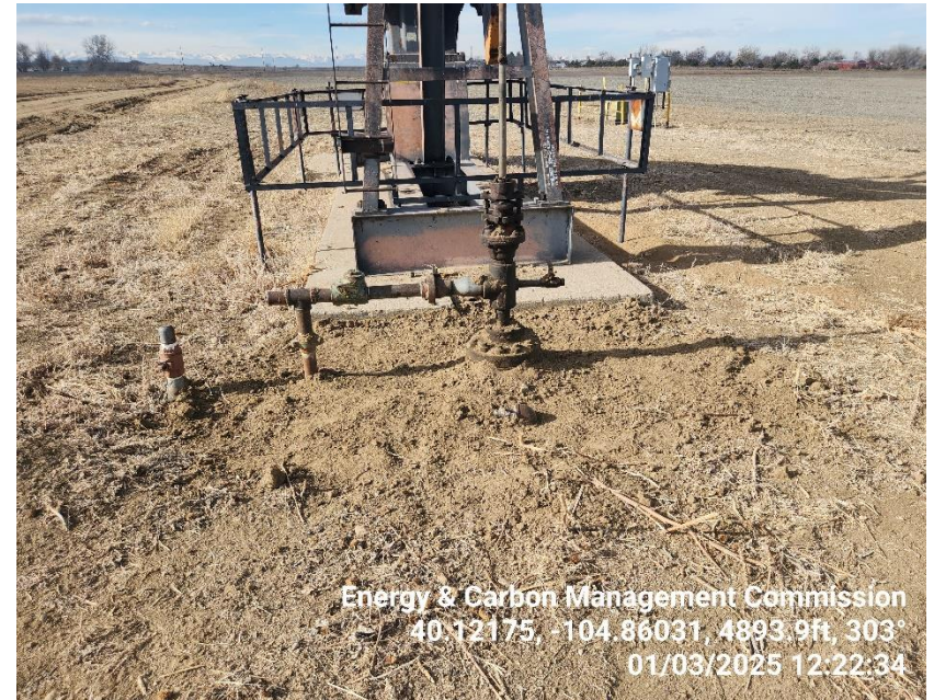
Photo 2 Stained material has been removed from around the Wellhead.
