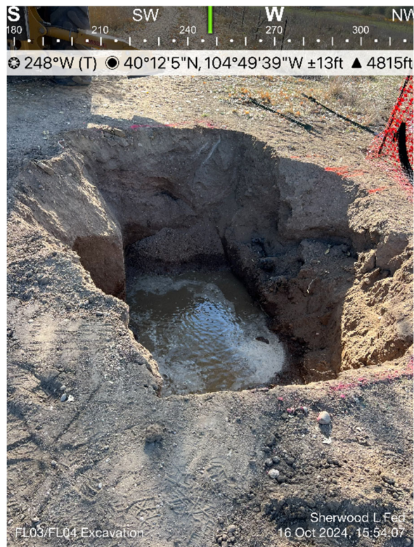
FL03/FL04 Excavation (Groundwater present)
