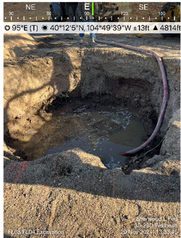
FL03/FL04 Excavation (Groundwater Present)
