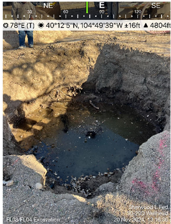
FL03/FL04 Excavation (Groundwater Present)
