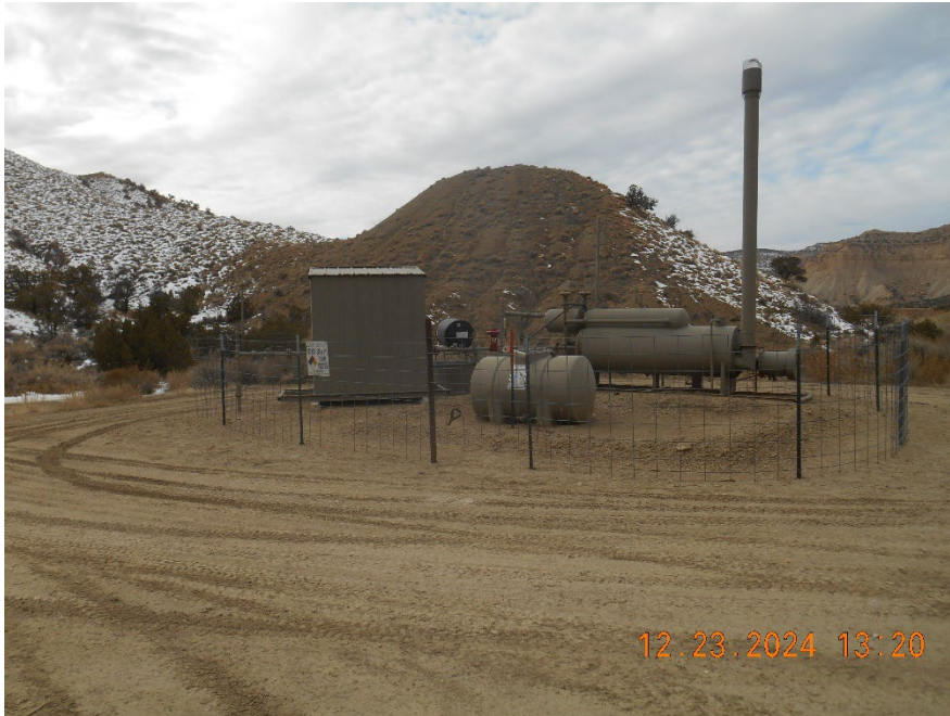
Separator and Meter housing
