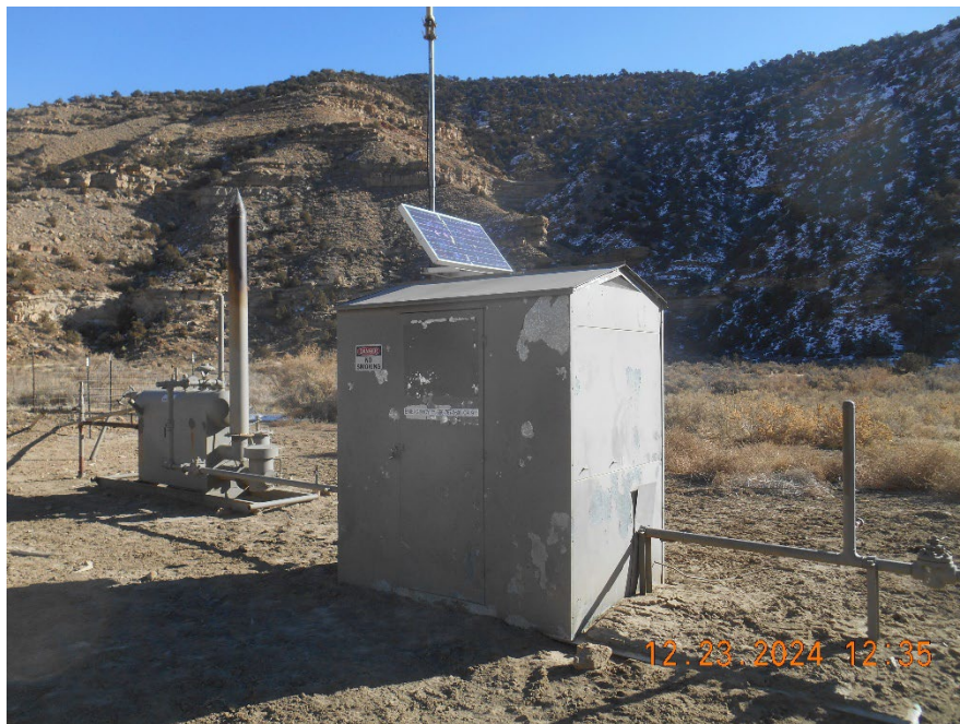
Separator and Meter housing
