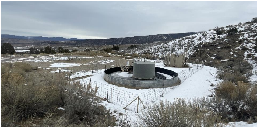
South West corner of location.
