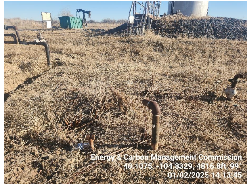
Photo 10 Unmarked flow lines.
