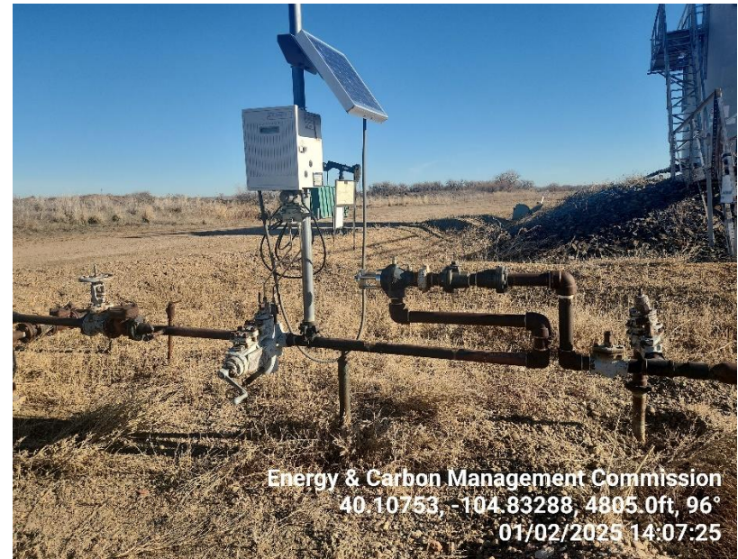
Photo 8 Gas meter run.
