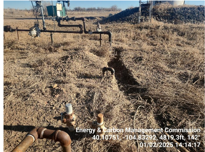
Photo 12 Unmarked flow lines.
