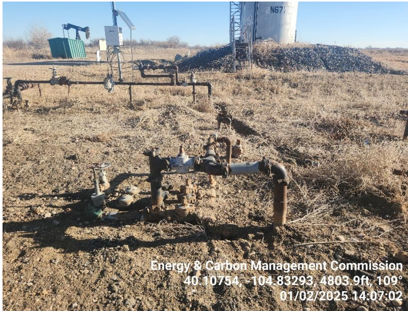
Photo 9 Flow line manifold.
