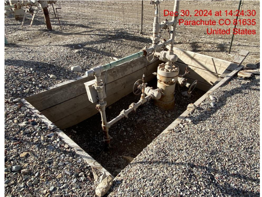
Open Wellhead Cellar – Photo #05665
