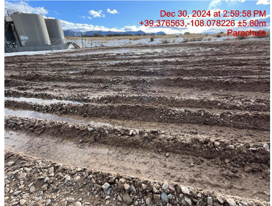
Photo # 1631 Lack of stabilization/compaction on location/insufficient BMP's
