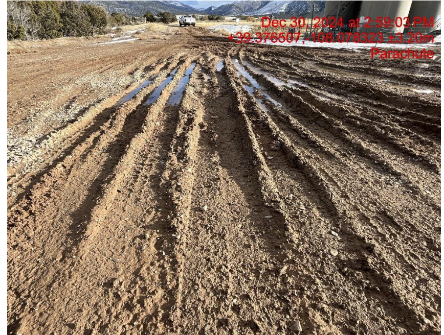
Photo # 1628 Lack of stabilization/compaction on location/insufficient BMP's
