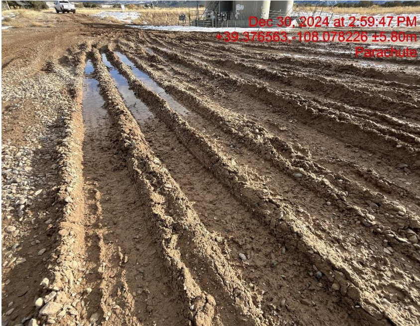
Photo # 1630 Lack of stabilization/compaction on location/insufficient BMP's
