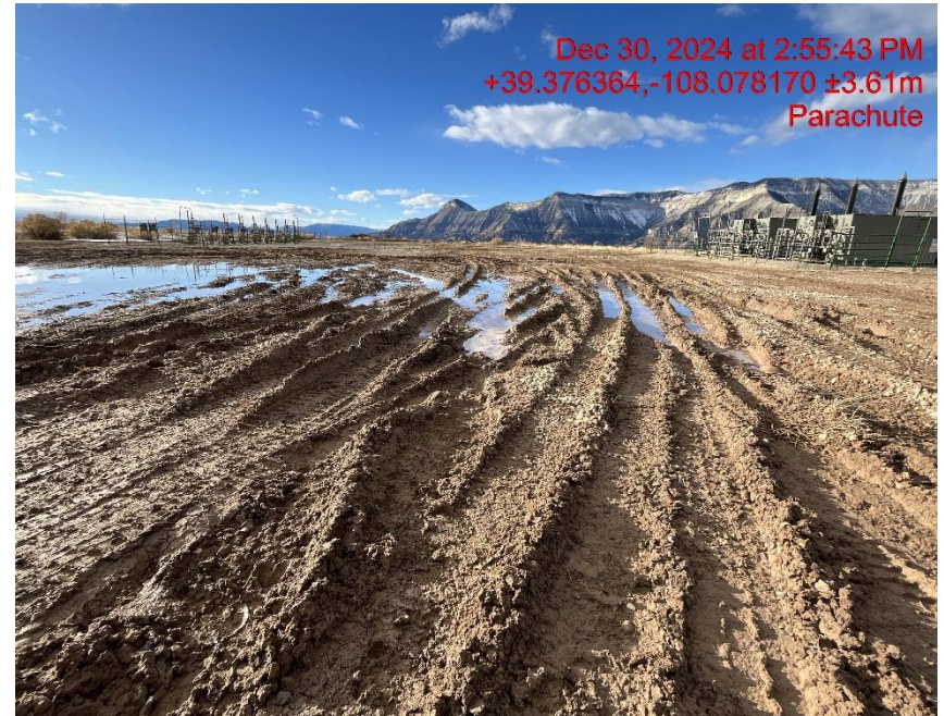
Photo # 1624 Lack of stabilization/compaction on location/insufficient BMP's
