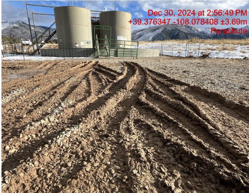
Photo # 1626 Lack of stabilization/compaction on location/insufficient BMP's
