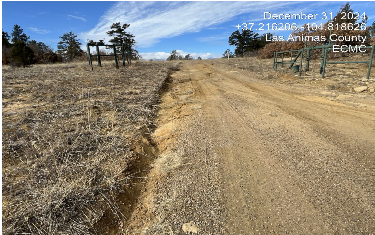
Photo 1. Facing northwest along the access road. This area has will need stormwater maintenance..
