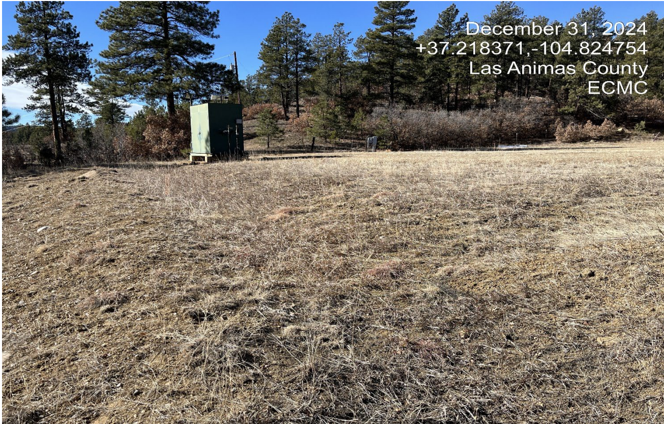
Photo 3. Facing southwest at the location.
