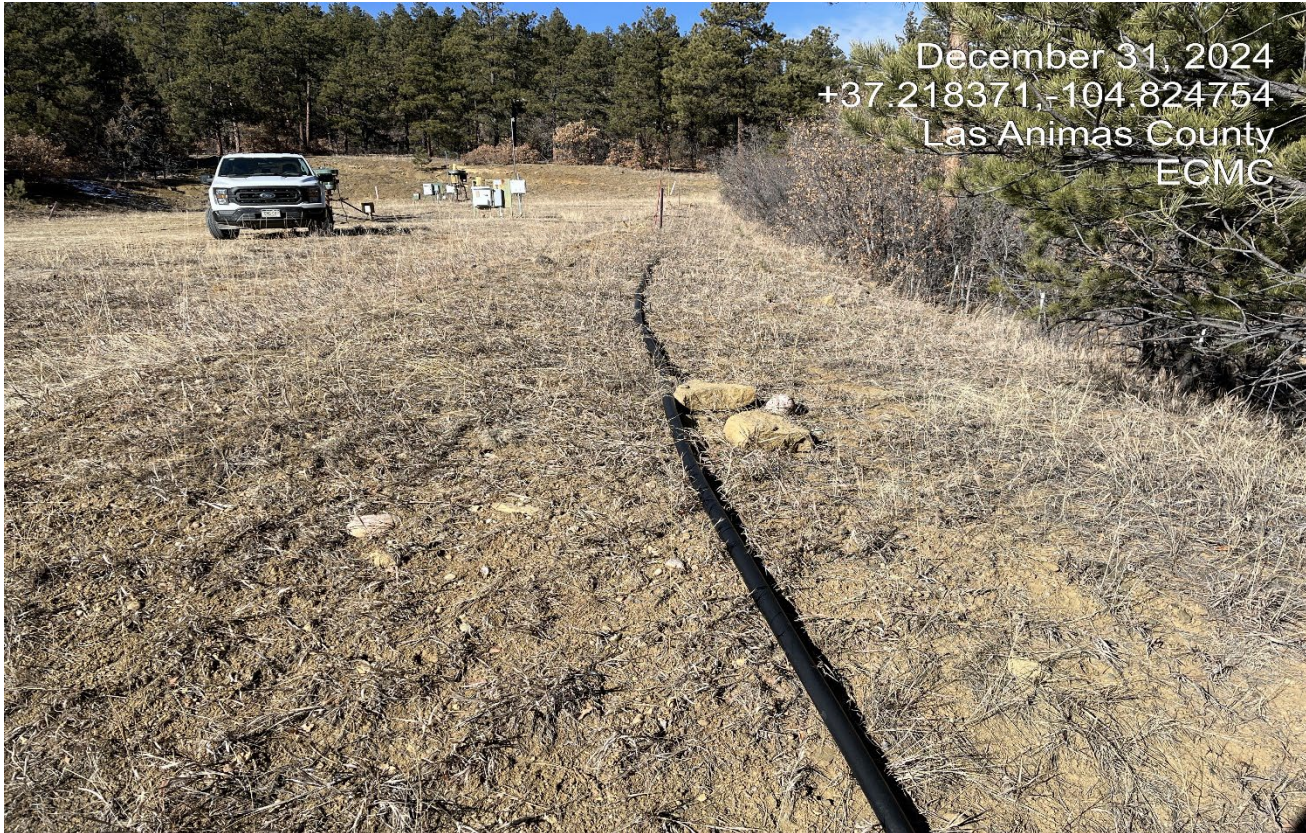
Photo 2. Facing west at the location. The black polyline transfers water to offsite pit.
