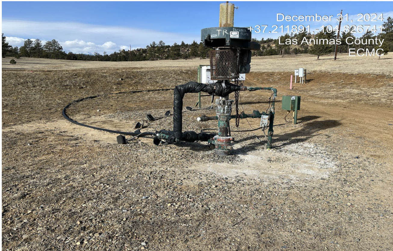
Photo 2. Facing toward the wellhead. There is whitened material around the wellhead possibly from a leaking wellhead.
