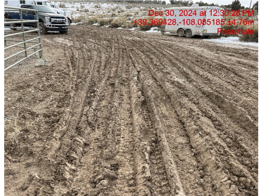
Photo # 1564 Lack of stabilization/compaction on location/insufficient BMP's
