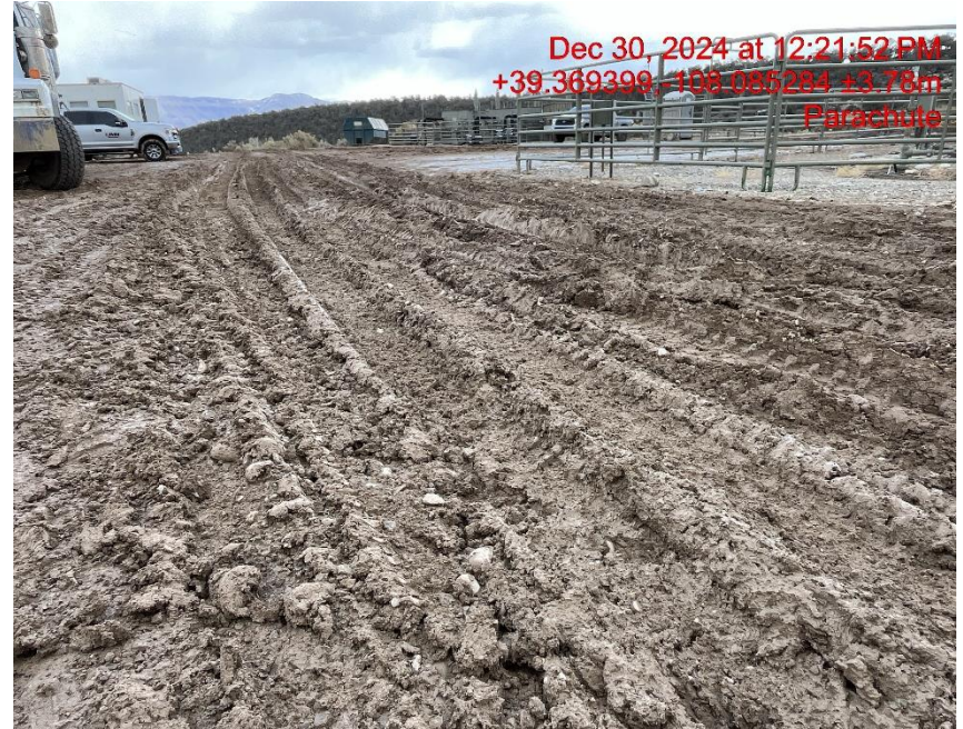
Photo # 1551 Lack of stabilization/compaction on location/insufficient BMP's
