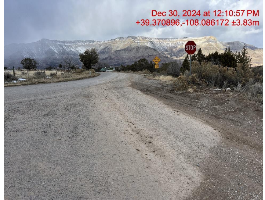
Photo # 1537 Tracking from lease road onto CR 306/Insufficient tracking BMP's
