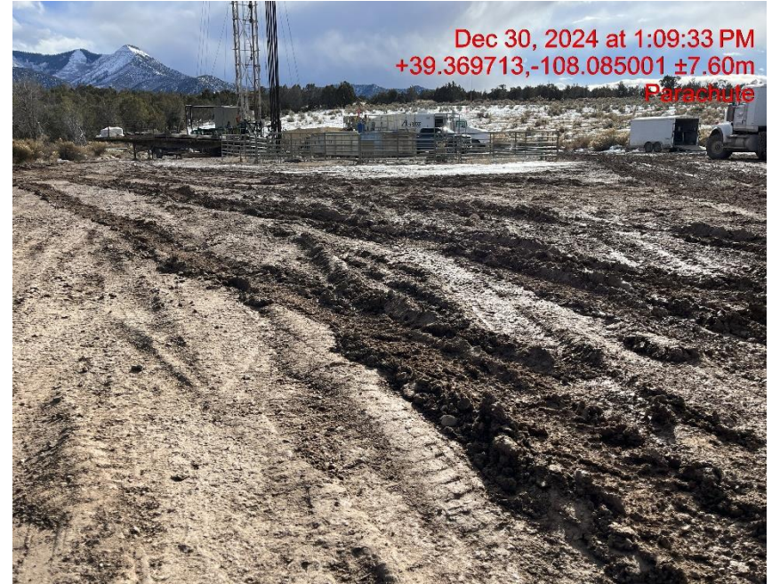
Photo # 1571 Lack of stabilization/compaction on location/insufficient BMP's
