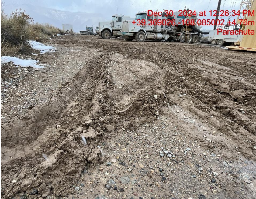
Photo # 1560 Lack of stabilization/compaction on location/insufficient BMP's
