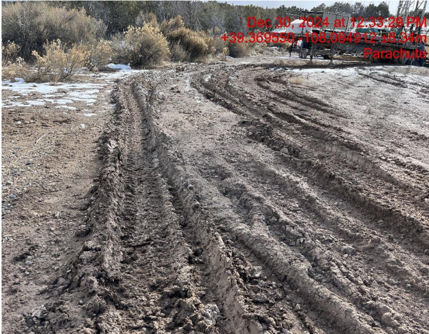
Photo # 1567 Lack of stabilization/compaction on location/insufficient BMP's
