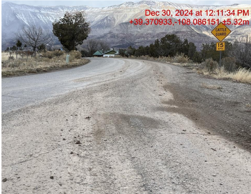
Photo # 1539 Tracking from lease road onto CR 306/Insufficient tracking BMP's
