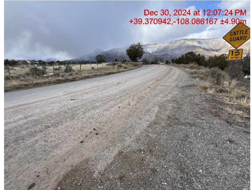
Photo # 1527 Tracking from lease road onto CR 306/Insufficient tracking BMP's
