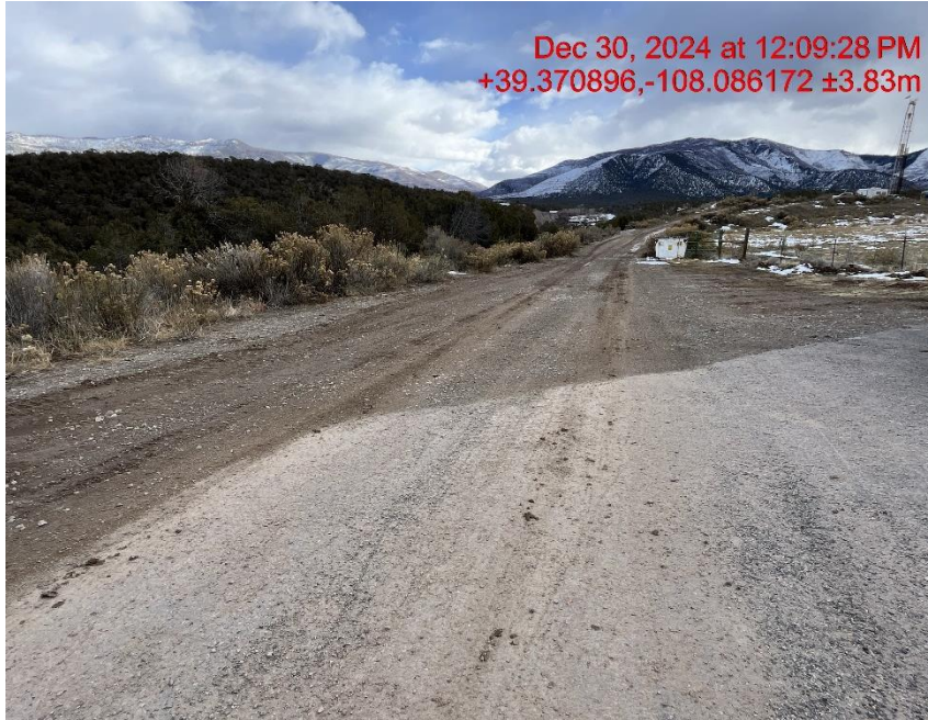
Photo # 1533 Tracking from lease road onto CR 306/Insufficient tracking BMP's
