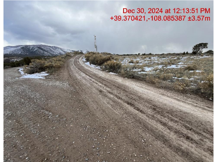
Photo # 1543 Tracking on lease road/Insufficient tracking BMP's
