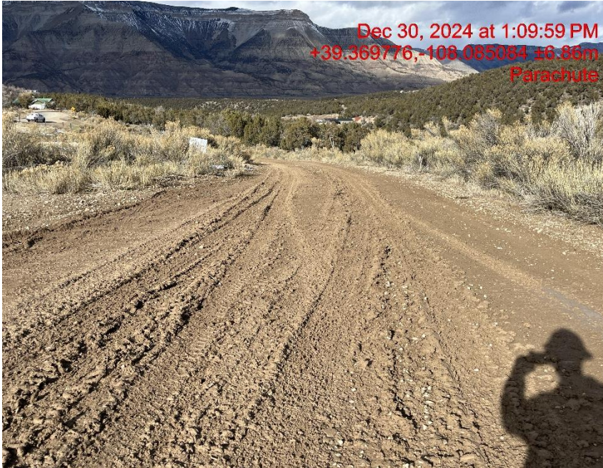
Photo # 1573 Lack of stabilization/Compaction/Insufficient tracking BMP's/Tracking from location onto lease road
