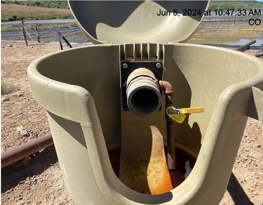
Photo # 9377 From inspection 708903976 conducted on 06/05/2024 Open ended load line
