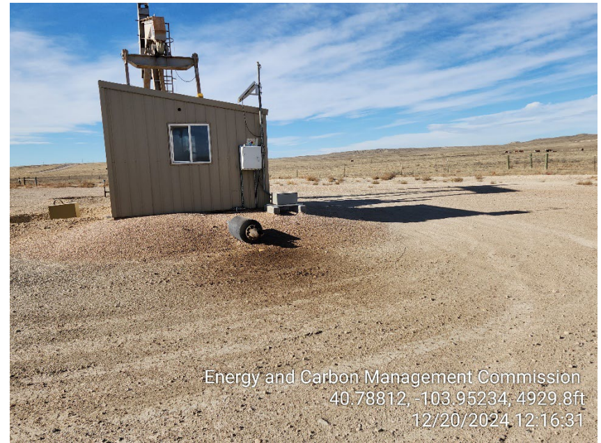
Photo 2 – Stained Soil at Engine Exhaust
