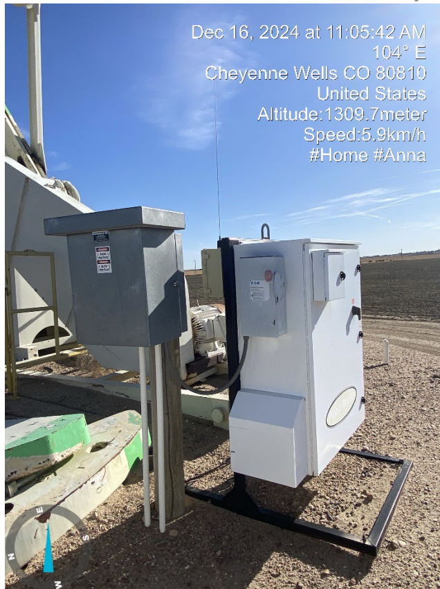
5. Elec panel, Cathodic Rectifier
