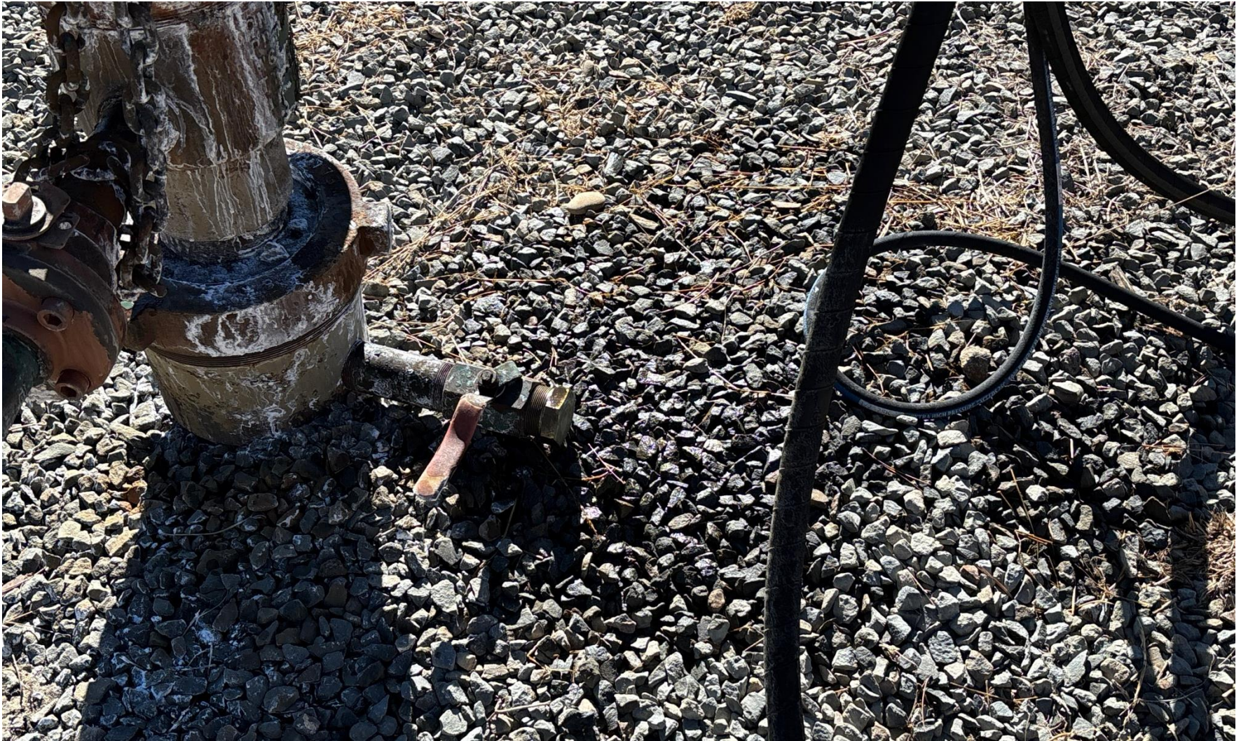
PHOTO 5: AREA OF IMPACTED SOIL UNDER LEAKING DRIVE MOTOR. Conduct maintenance on equipment, cleanup stained material and review self inspection processes. COMPLY WITH RULE 1002,.(2).D. CA DATE 1-9-25
