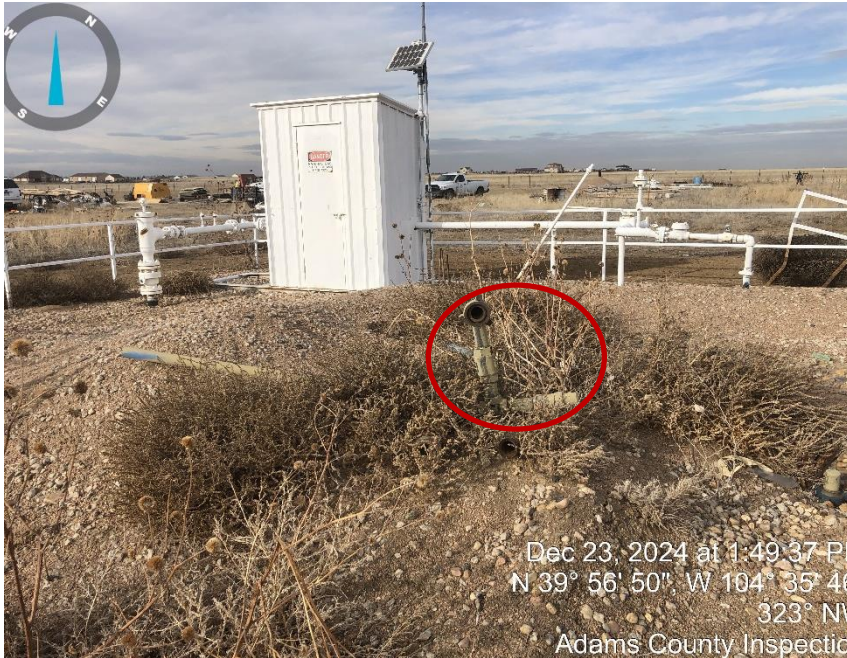
Photo #5 Meter, unmarked risers & weeds.
