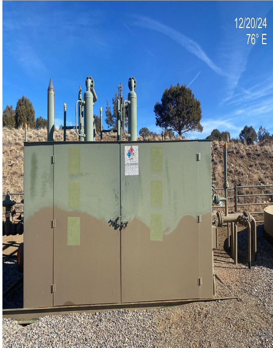
Photo 4. Separator and Produced water tank signs/placards are starting to deteriorate, future maintenance is advised.
