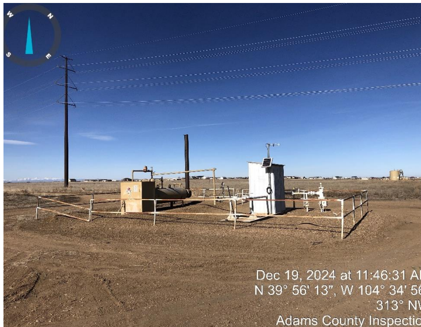
Photo #3 Separator & Meter.
