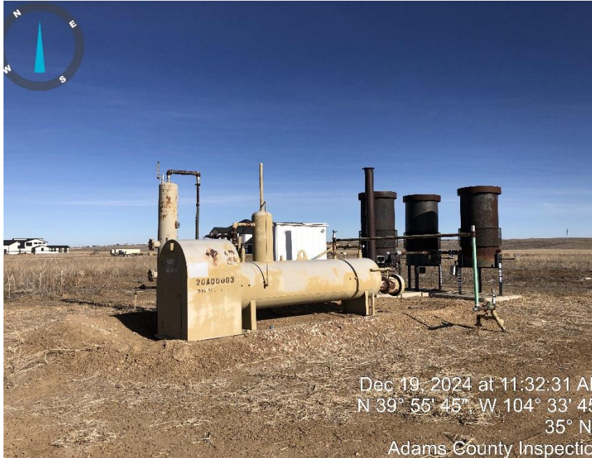
Photo #3 Separator, ECDs & Meter.
