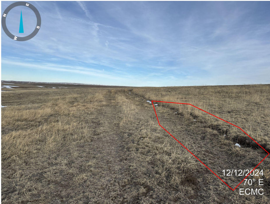
Photo 1. Photo taken Looking east along access road. Desirable vegetation coverage is progressing. Isolated areas may need recontouring or topsoil filling.
