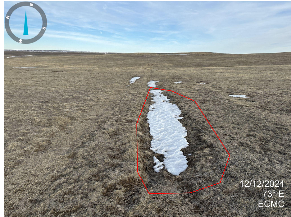
Photo 2. Access road looking east. Access road appears to be reclaimed except for two areas that may need to be filled and stabilized. See Photo 1.
