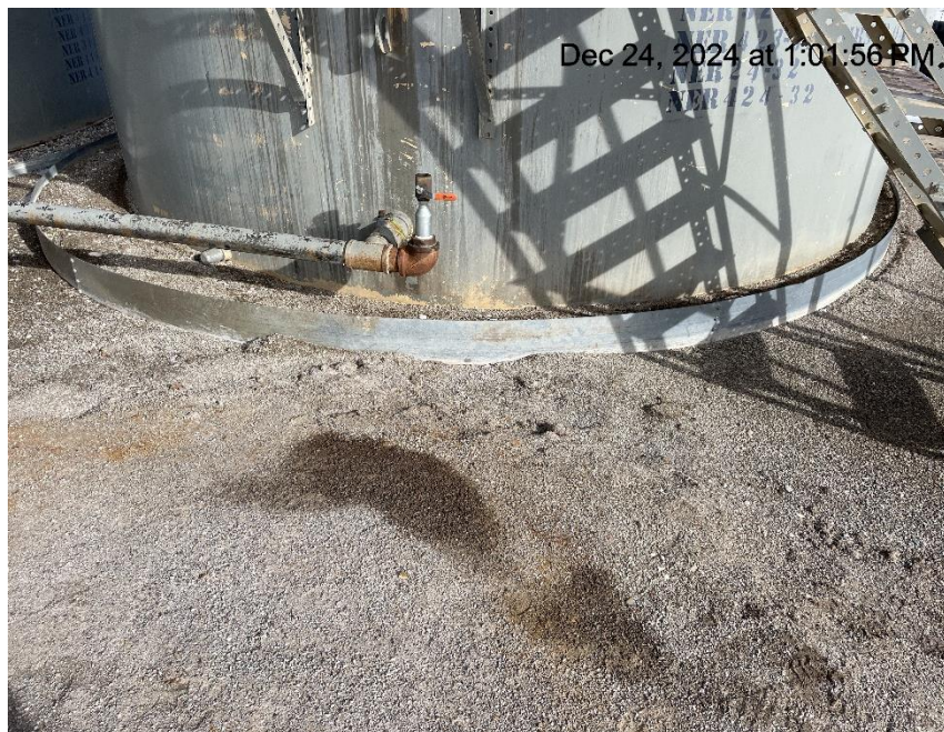
Photo # 5432 Staining in secondary containment
