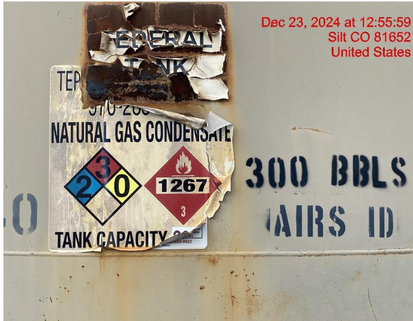
Weathered Tank Label Needs Replaced – Photo #05556
