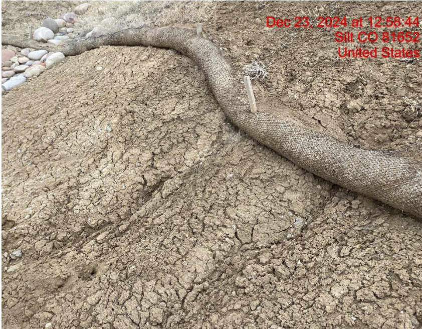
Rill Erosion Undercutting BMP – Photo #05564
