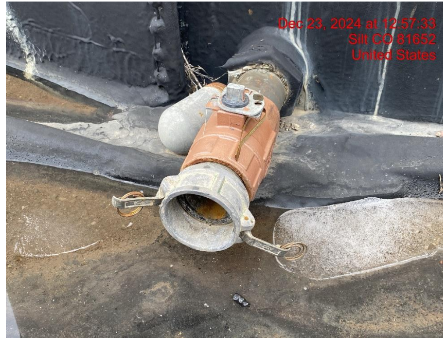
Open-Ended Line on Tank – Photo #05559
