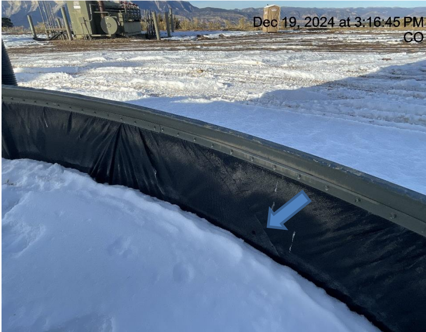
Photo # 4744 Hole in liner/liner needs maintenance
