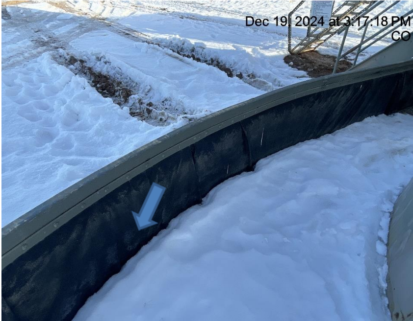
Photo # 4746 Hole in liner/liner needs maintenance
