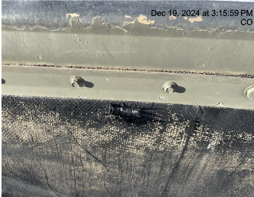
Photo # 4740 Hole in liner/liner needs maintenance
