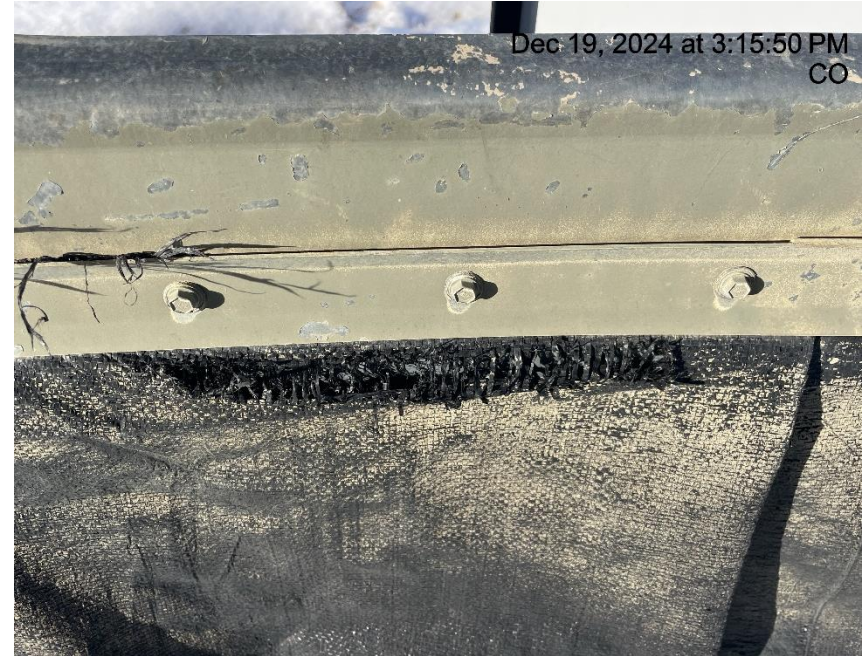
Photo # 4741 Hole in liner/liner needs maintenance
