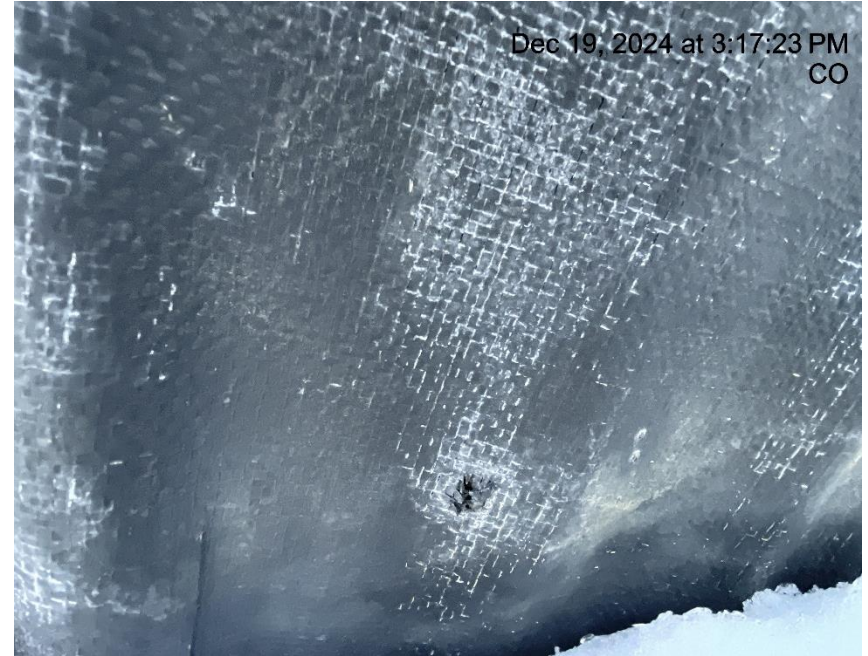
Photo # 4747 Hole in liner/liner needs maintenance
