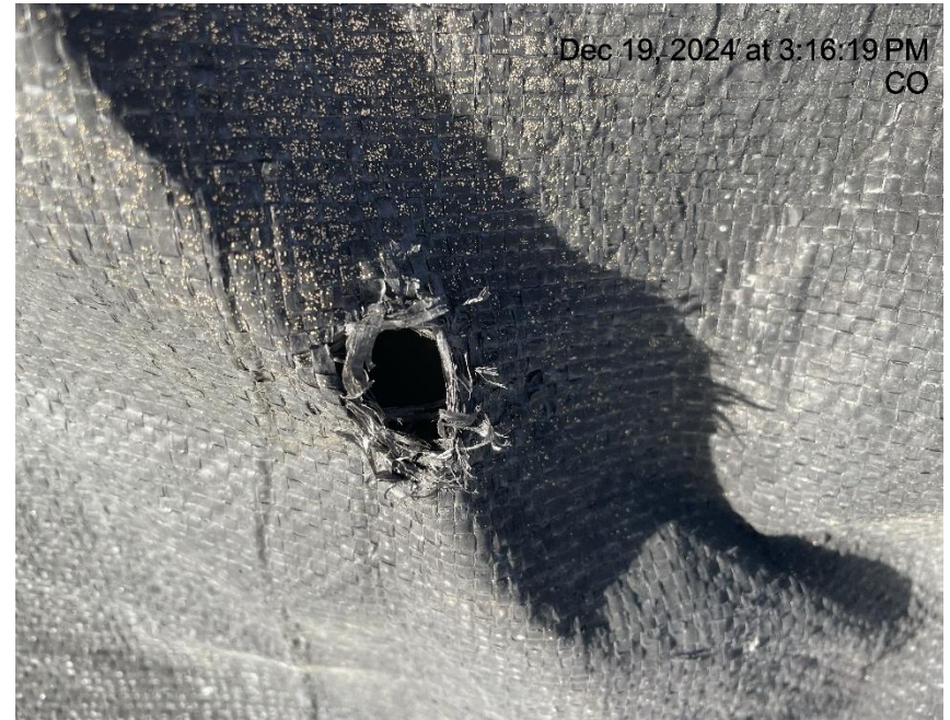
Photo # 4743 Hole in liner/liner needs maintenance
