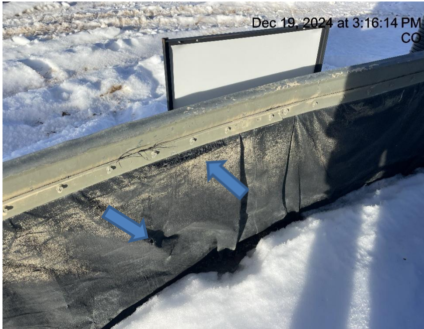
Photo # 4742 Holes in liner/liner needs maintenance
