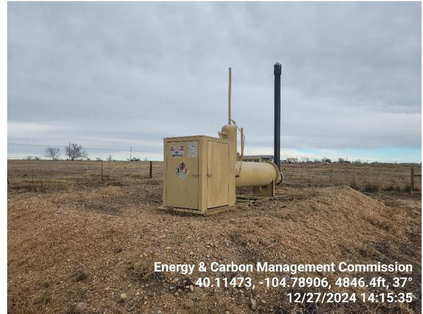
**Photo 10 Heated Horizontal Separator.**
