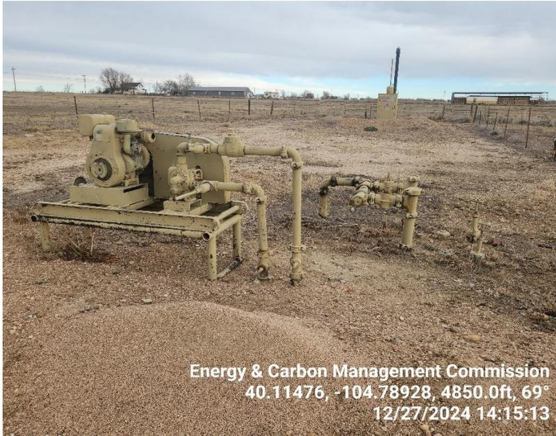
**Photo 9 Flow line manifold.**
