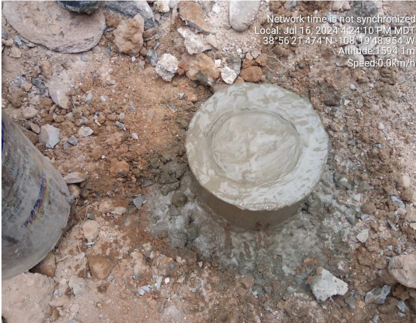
Cement to surface.
