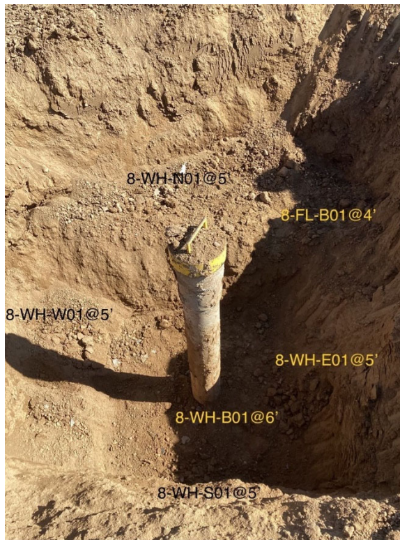
Wellhead Excavation
