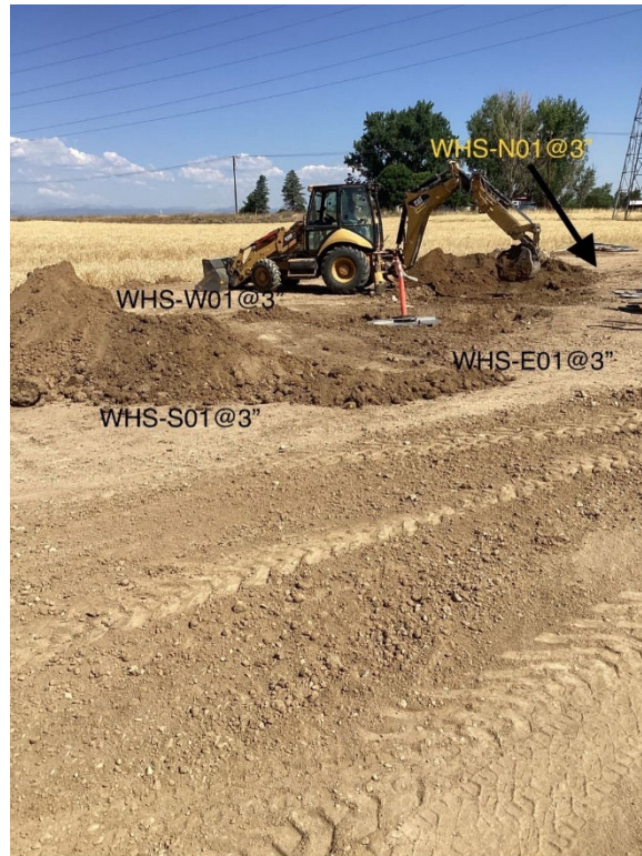
Wellhead Excavation
