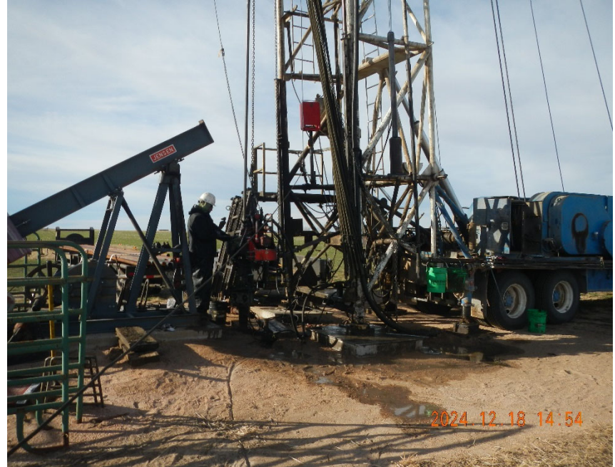
4. Crew at work hydro testing tubing string.
