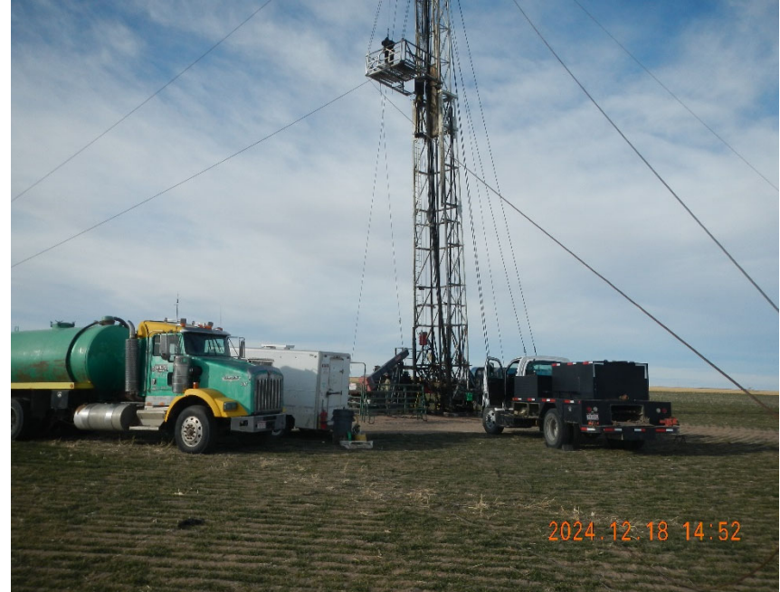
2. View of equipment on site for well workover.
