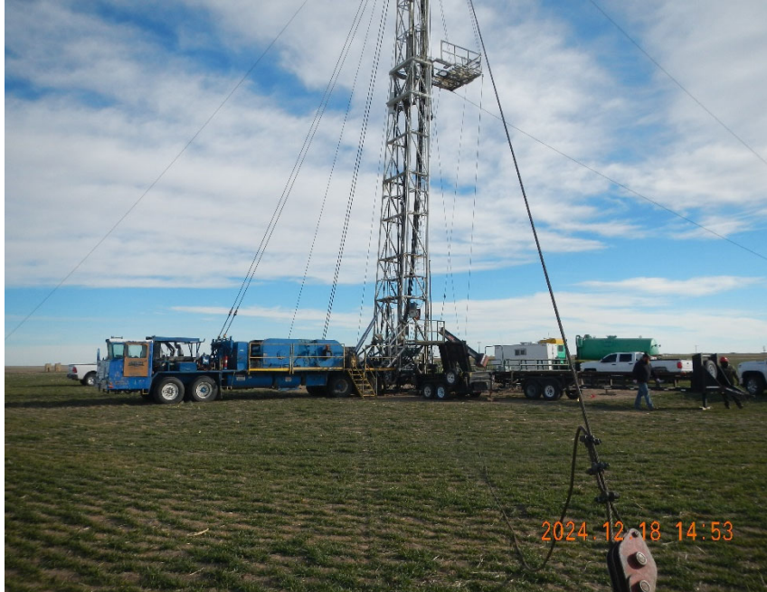
3. View of well location.
