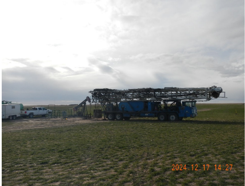
4. Rig spotted in over wellbore for workover.
