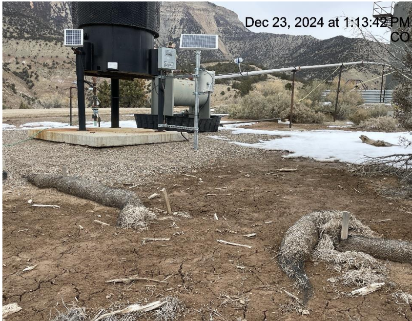
Photo # 5096 Wattles damaged/need maintenance
