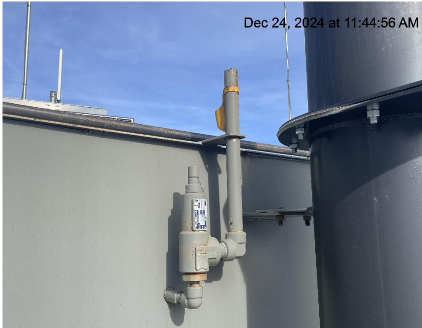
Photo # 5277 PRV vent line does not comply with CECMC pressure safety device rules
