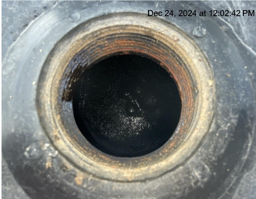
Photo # 5283 Failure to maintain chemical BMP - Chemical tank containment approximately 2/3 to 3/4 full of fluid/BMP insufficient to contain possible spill
