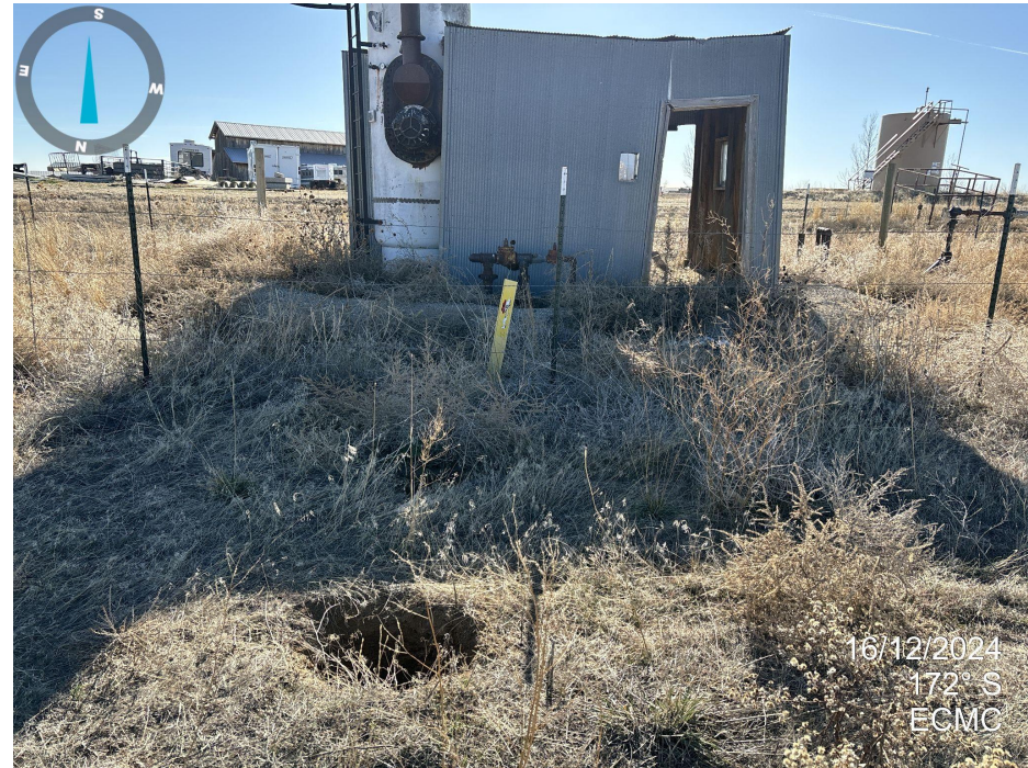
Photo 8. Pothole near tank battery. Approximately 2 ft deep.
