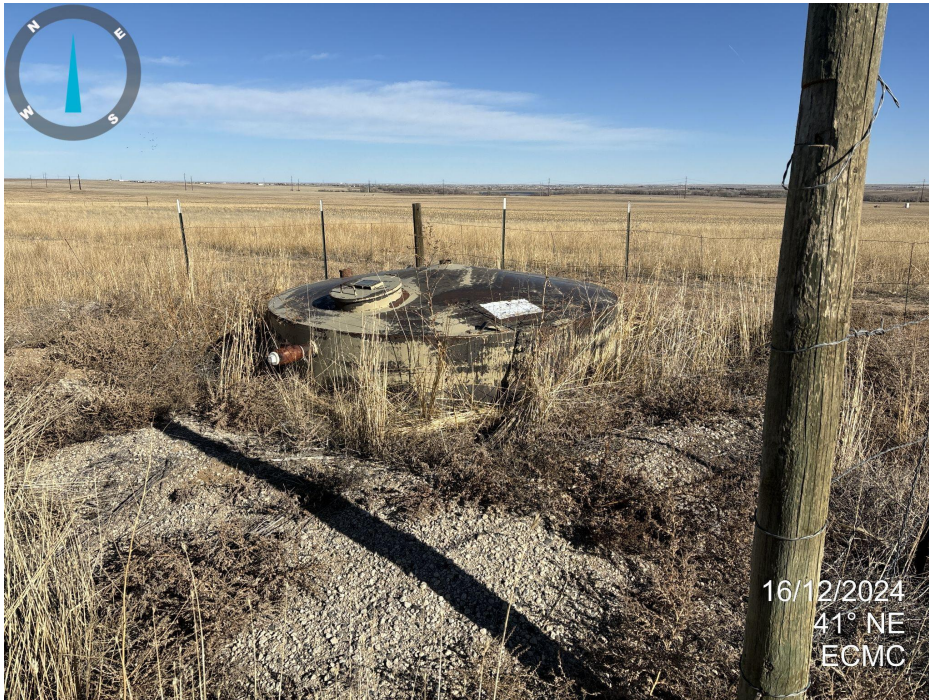
Photo 3. Looking at east side of tank battery. Partially buried vessels sign is degraded and cap is removed allowing wildlife access.
