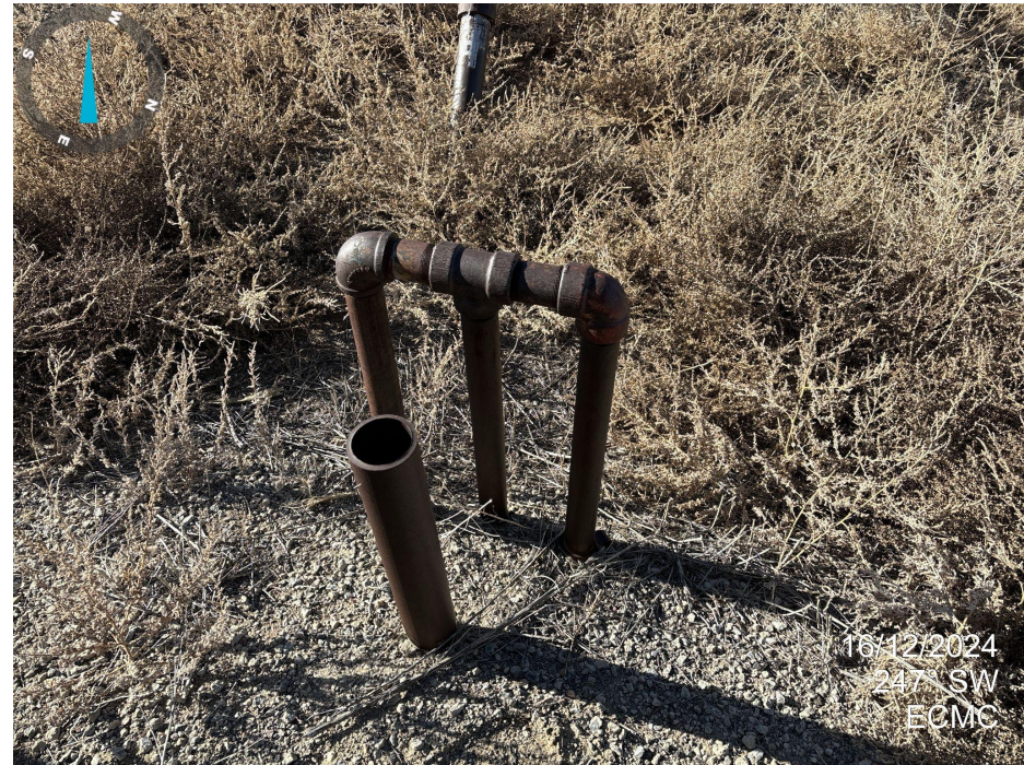
Photo 6. Uncapped pipe at tank battery location.
