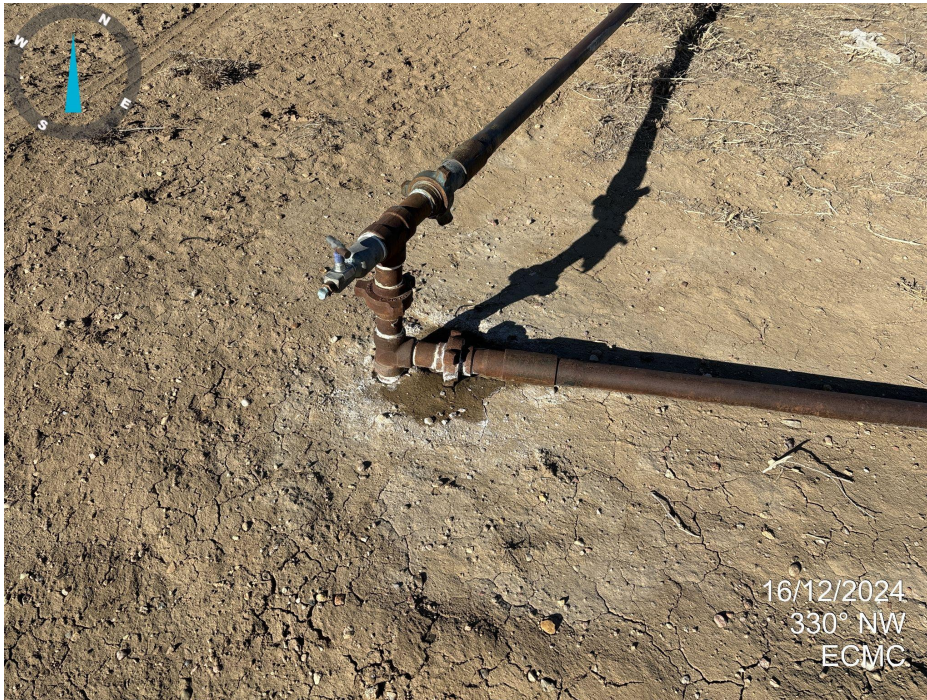
Photo 5. Stained soil at joint between produced water tank and separator.
