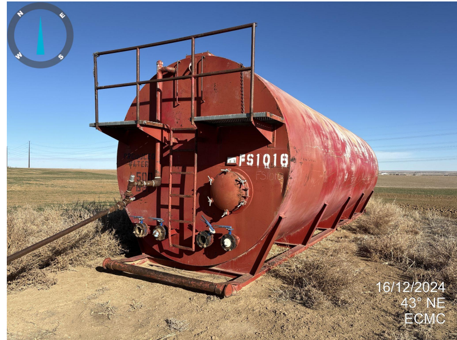
Photo 6. Produced water tank with no secondary containment.
