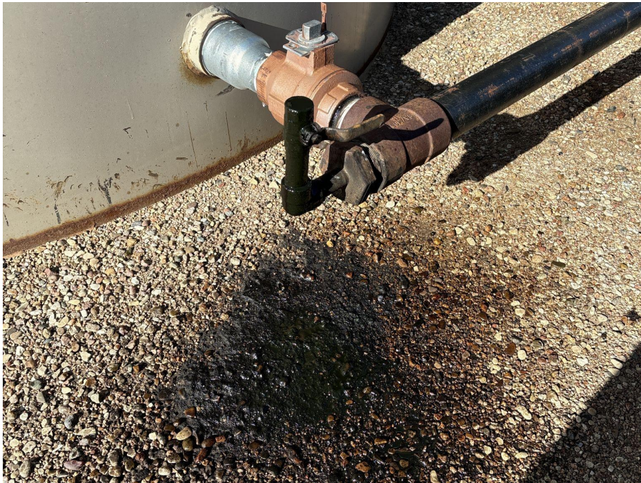
Photo 3. Southernmost crude oil tank has a leaking valve and stained soil beneath it in secondary containment.
