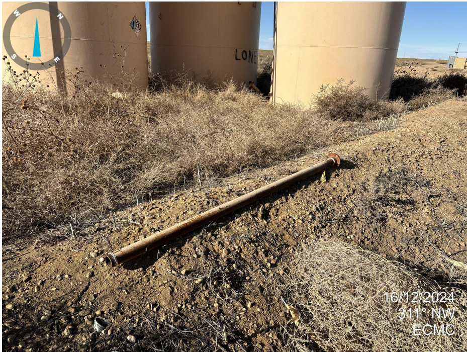
Photo 4. Looking northwest at tank battery. Unmanaged weeds in secondary containment. Unused equipment remains on site.
