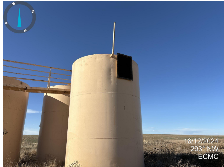
Photo 5. Eastern tank has an open inspection hatch.
