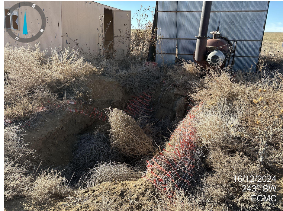
Photo 7. Approximate 6'x10'x4' hole dug behind separator. Degraded construction fence remains but does not restrict access.
