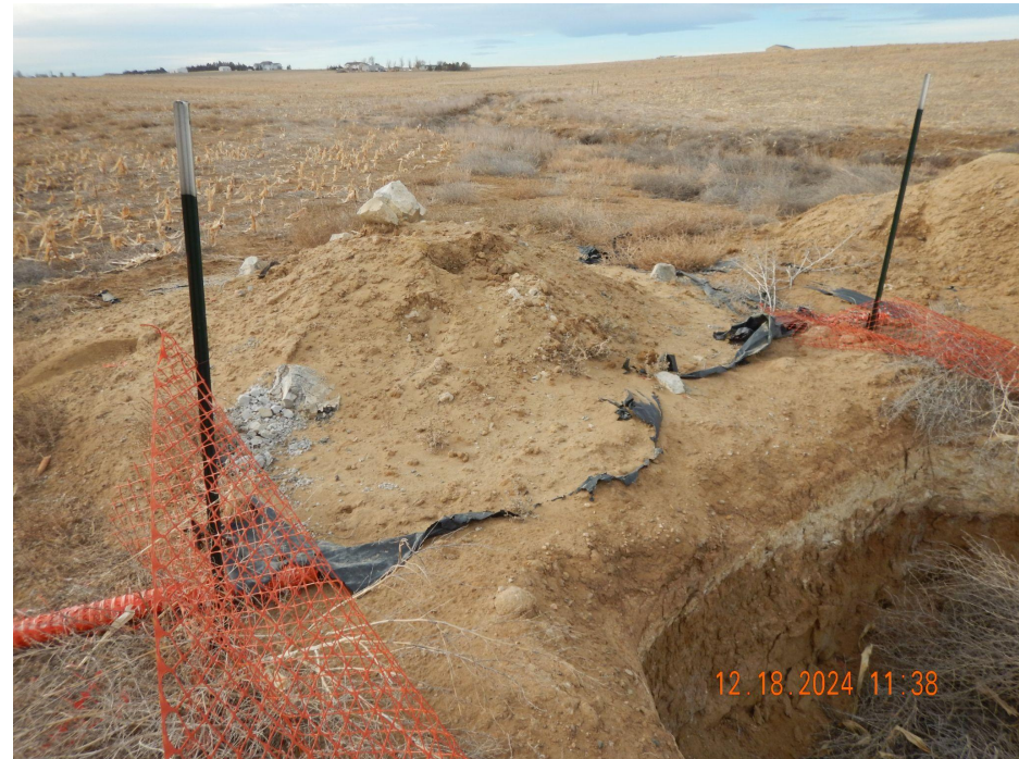
Photo 3. Soil has been placed on liners without proper stormwater BMPs. Concrete debris and trash are present.
