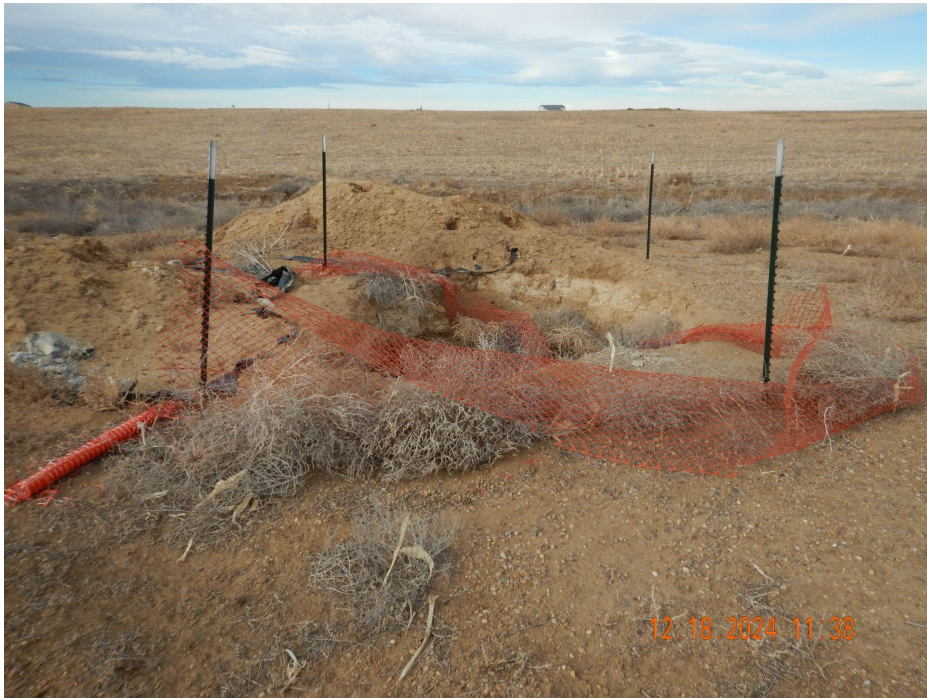
Photo 2. Looking across the wellsite. Well appears to be plugged and abandoned. Open excavation with improperly installed fences.
