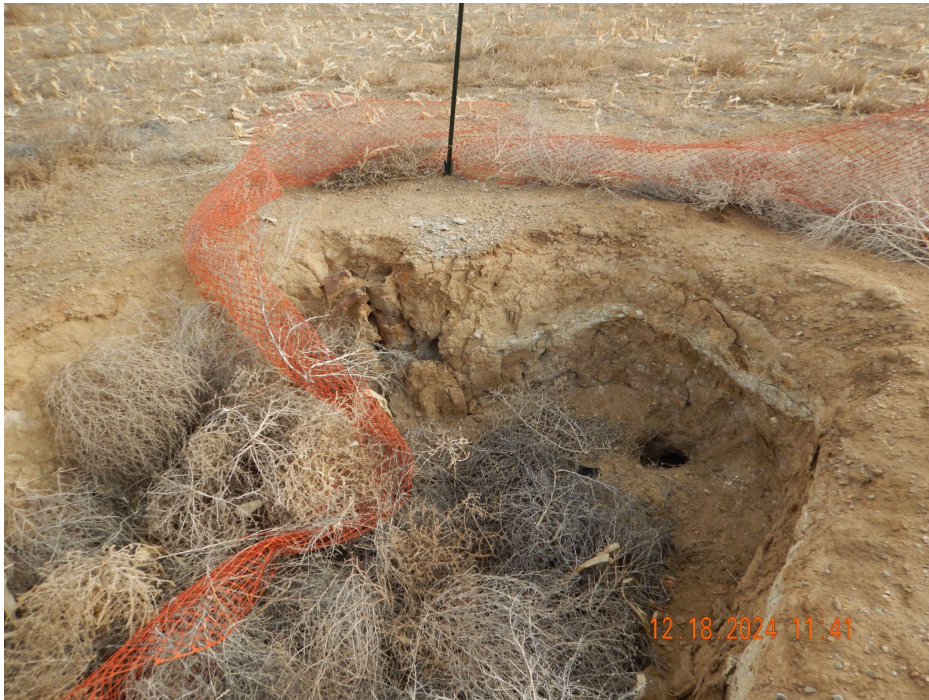
Photo 4. Debris (tumbleweed) is present within the excavation. Metal pipe, possibly the well head is visible.
