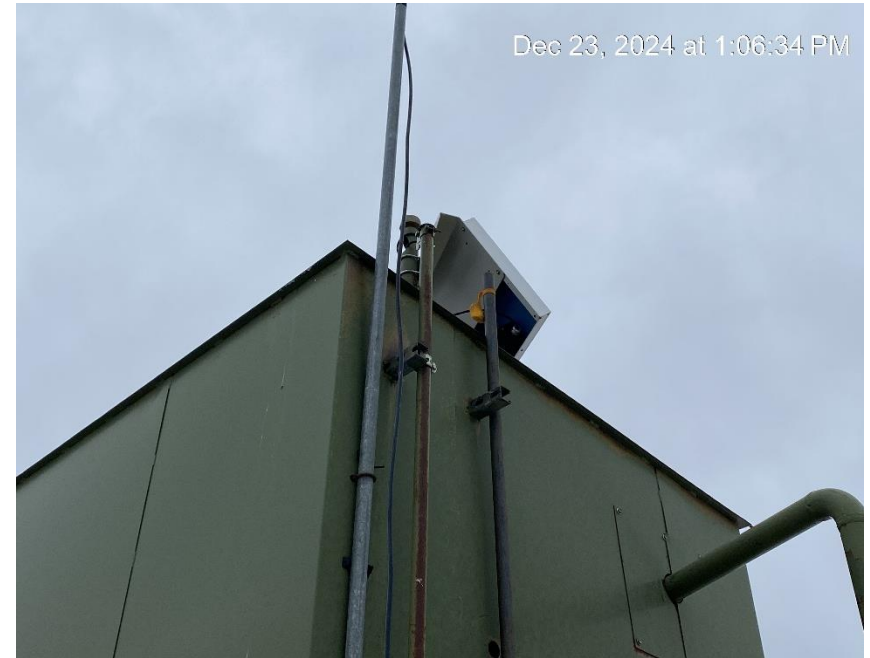
Cap off vent relief riser
